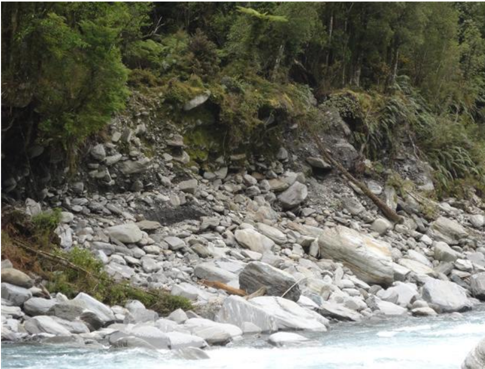
Figure 3: The Waitaha left bank opposite the powerhouse site.
